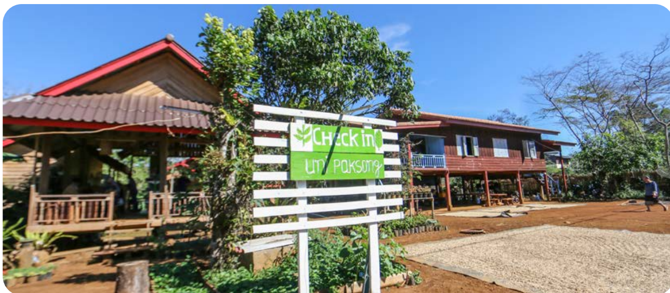
Photo: (CC BY-NC-ND 2.0) Asian Development Bank, The Paksong District coffee growers farmers cooperative store front entrance.jpg
