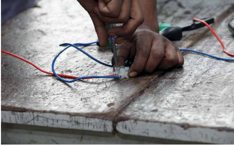
Replacement of splice joints with wire connectors significantly reduces electrical-fire risk (©Sarika Gulati, SEEDS)
