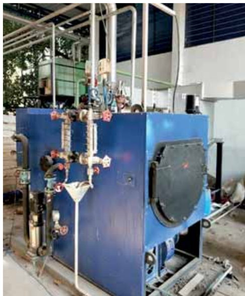
Biomass briquette boiler installed at AGL in FY 2019 (©ABFRL)
