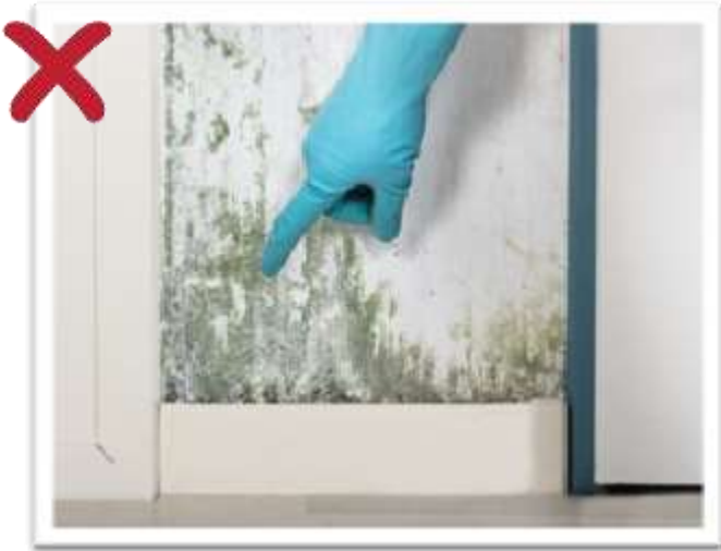
Figure 21: Fungal growth (moss) on walls can release toxic spores and contaminate food.
