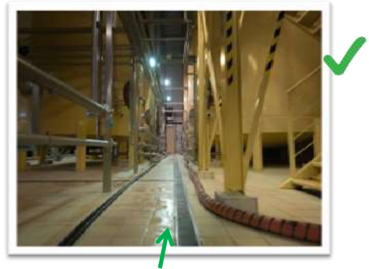
Figure 22: Floors should allow adequate drainage and cleaning.
