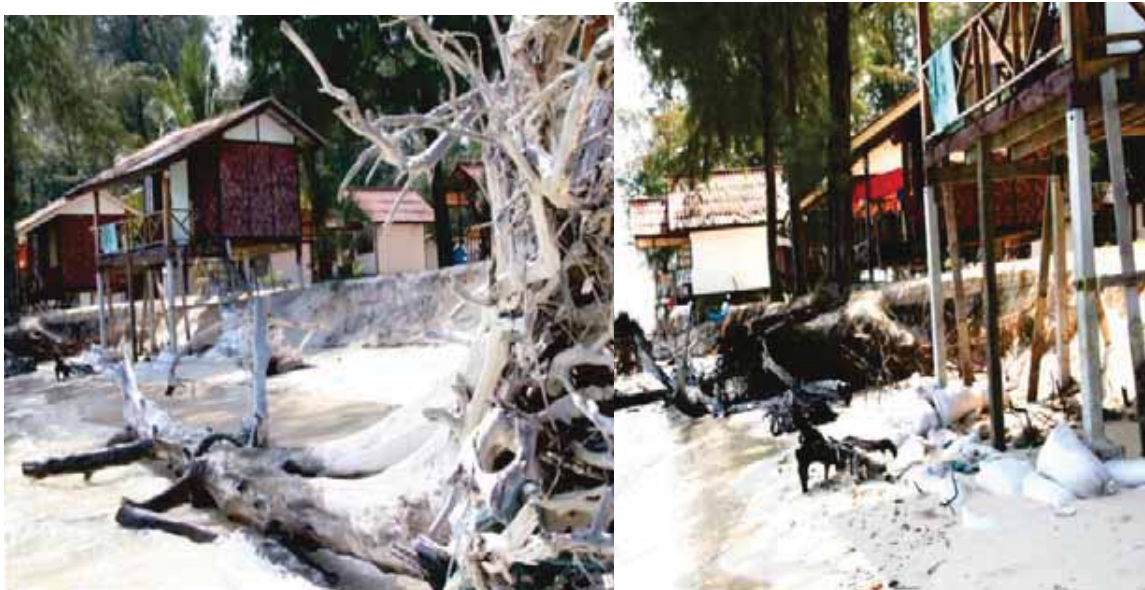
Plate 10. Severe erosion of a beach resort, Andaman Coast, Thailand
