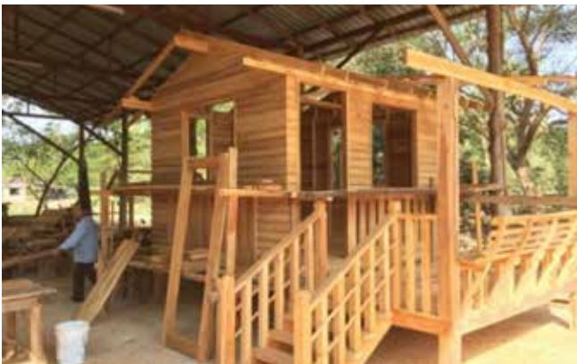
Prefabricated wooden cottage in Thailand (© Peter Viehbeck)
