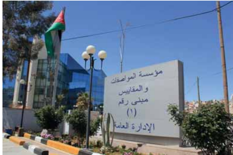
Headquarters of Jordan Standards and Metrology Organization (JSMO)
